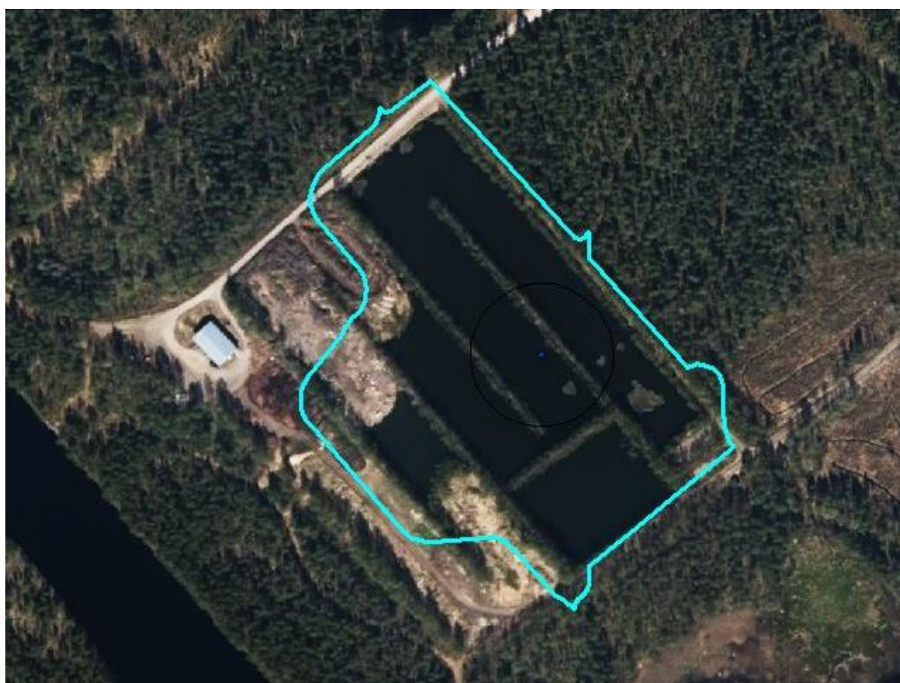
Wrong class: 1113 (a waste water treatment plant)
